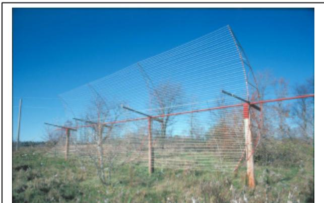
FIG. 2--One of the completed 5 X 15-metre antennas (autumn, 1986). The operating frequency is 238 MHz. (*Photograph by Frank Roy*).
